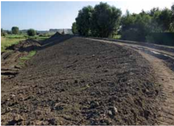
Figure 72. Earthworks: raising and widening the ring dyke
