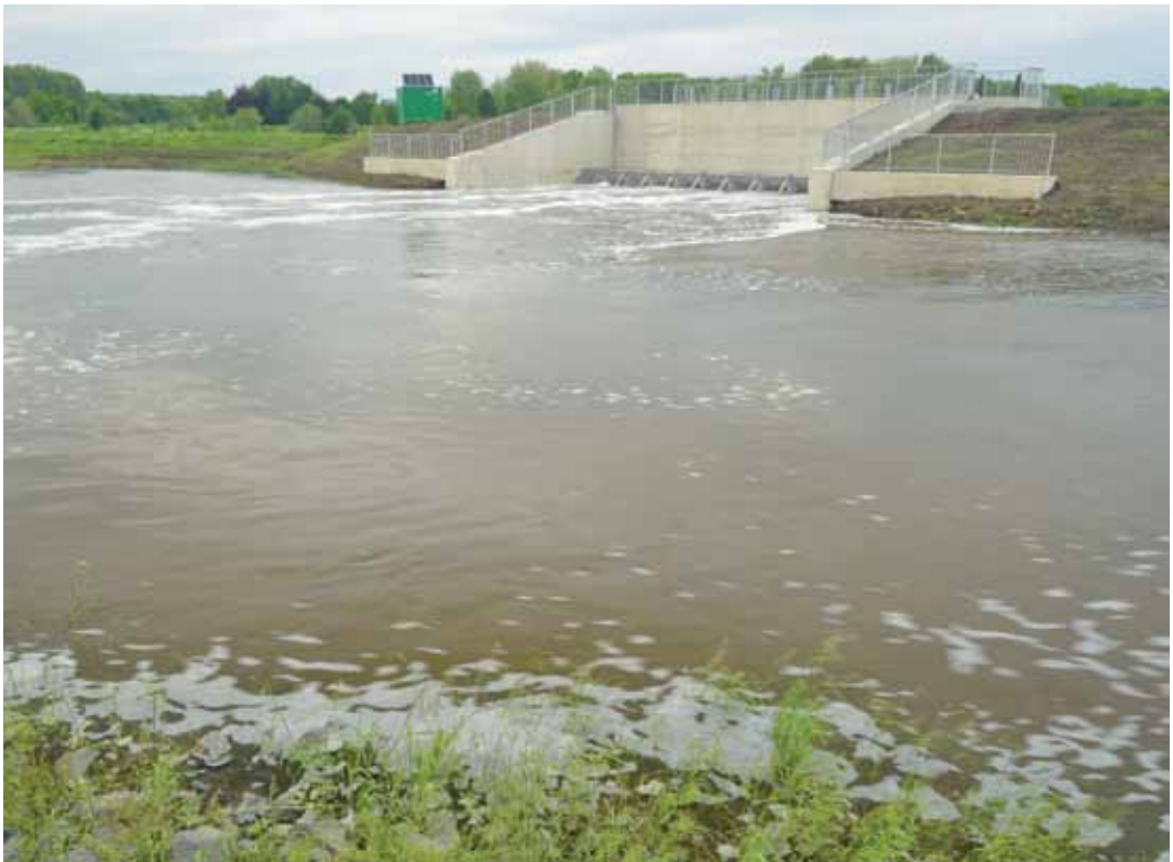
Figure 7.14. A completed FCA-CRT
