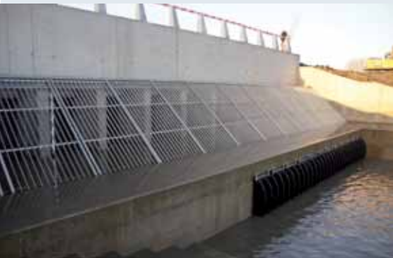
Figure 7.10. Installation of the framework infrastructure
