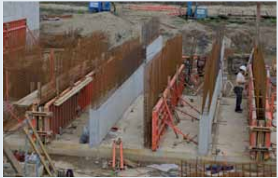
Figure 7.7. Concreting the walls
