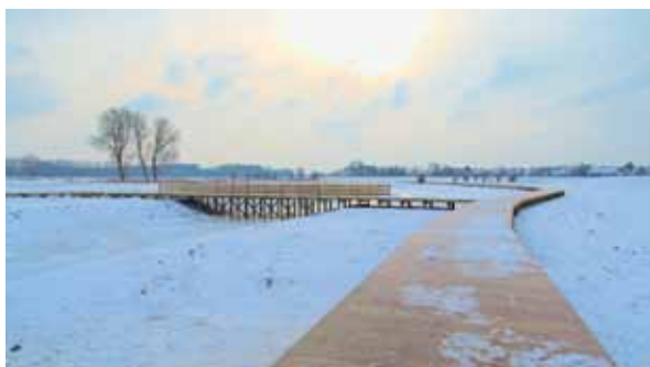
Figure 7.13. Start of the walkway
