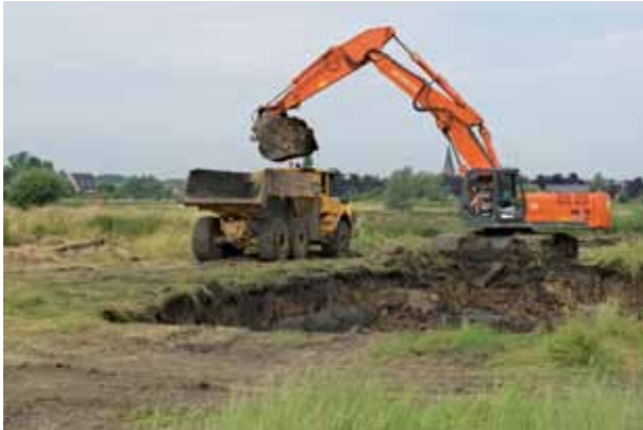
Figure 71. Earthworks: start of excavating the channel source
