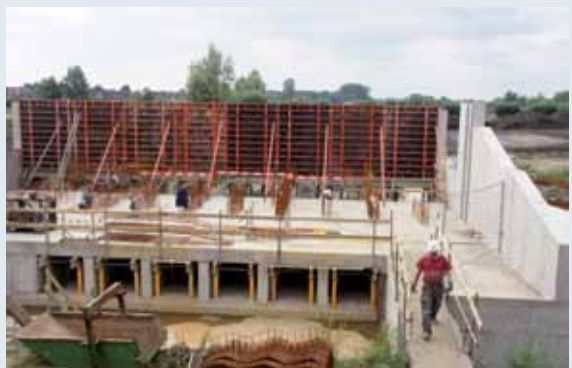
Figure 7.9. Formwork and reinforcement of the superstructure
