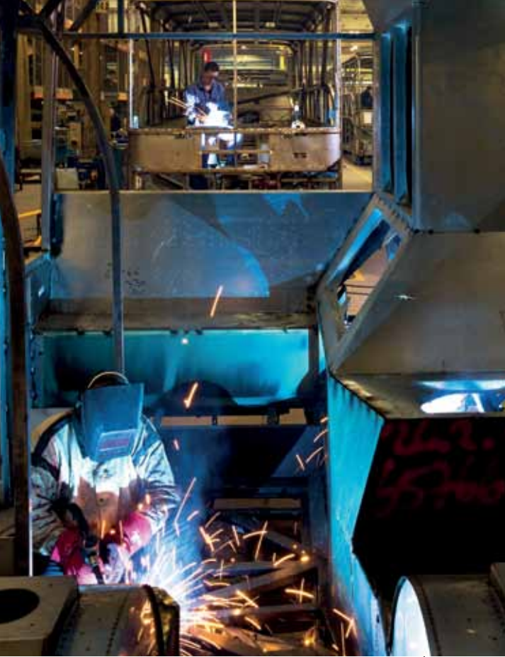
Welders at work at the construction atelier for busses - Van Hool, Koningshooikt © Tom Dhaenens
