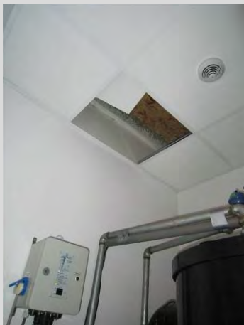
Berging die later liftschacht kan worden. KiDs vzw, © Inter
