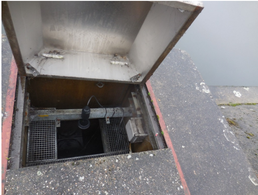
Figuur 5 – Peilput Vega radar
