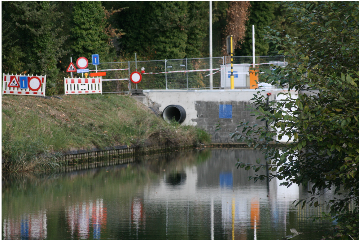
Figure 2 – View of the drainage structure from Lock No. 3 in Dessel-Schoten.
