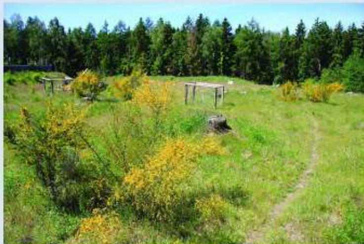
Figure 29.5 Wildlife overpass for mammals, reptiles, amphibians and invertebrates in Germany. Designed to maximise habitat heterogeneity, this structure has three different soil types and ponds on both approach ramps and includes grassy and shrubby vegetation. A range of invertebrate species can use the bridge, including those preferring drier or moister environments and those that prefer grasses or shrubs. The two wire enclosures are part of an experiment to test the effect of ungulates on plant growth. Source: Photograph by H. Reck.
