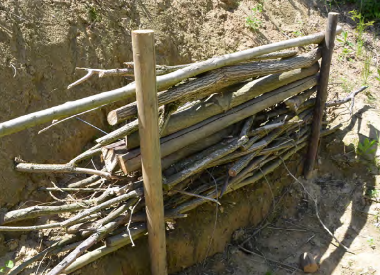
dastunnel in Opvelp
