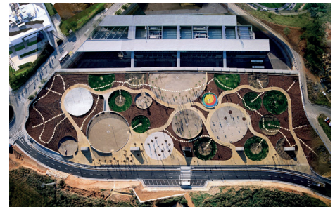
DAKPARK OP DE BUSDEPOT - HORTA BUS DEPOT, BARCELONA - DFT ARCHITECTS
