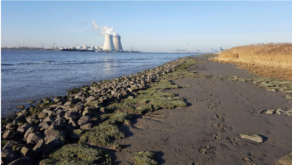
Figure 2.2 Boundary between the marsh and tidal flats at Galgeschoor with the presence of the riprap ridge
