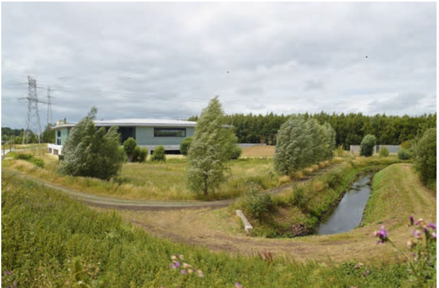
OO 2106 Crematorium, Zemst, Christian Kieckens Architects - DAE, 2015
