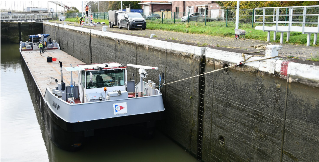
Figure 6 - Zulu 1 positioned in lock chamber during PoC Iv-Infra
