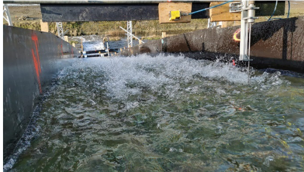
Figure 18 – Ultrasonic water level and electromagnetic point velocity meter mounted on small upper portal
