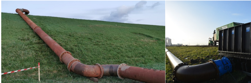
Figure 3 – Steel tube system right: pressurized entrance to dissipation box
