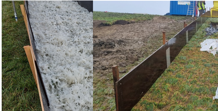
Figure 9 – Side boardings (left overflow tests, right: INFRAM overtopping tests)
