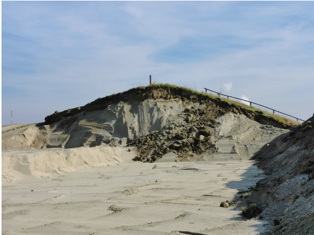
Figure 33 - Internal structure of the levee near N-OF05 during excavation. The clay cover layer is less approx. 80 to 100 cm thick.
