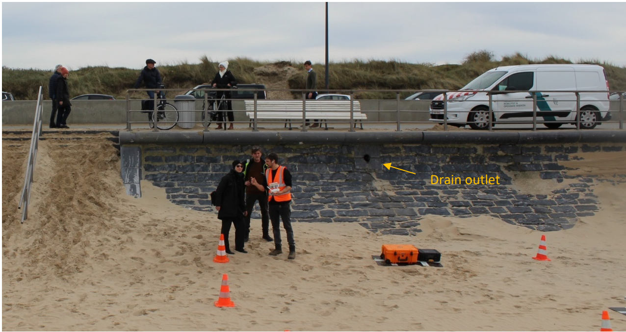
Figure 11 – The seawall in Raversijde, after the excavation works. Notice the drain outlet
