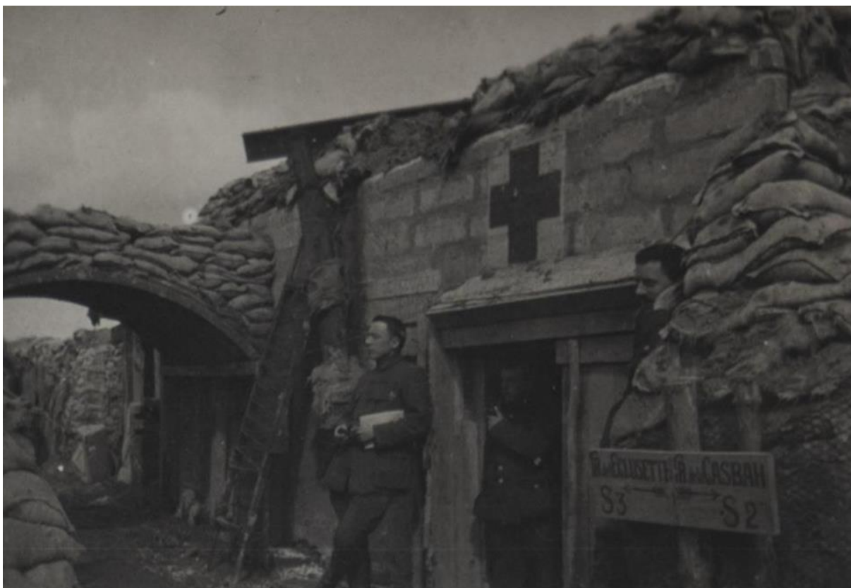
Figuur 10 Tranchée de l'Eclusette (bron: In Flanders Fields Museum , IFFFA001_000005-3)
