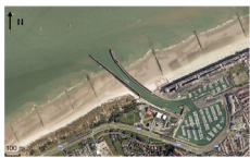
Figure 1 Beaches and harbor entrance of Blankenberge
