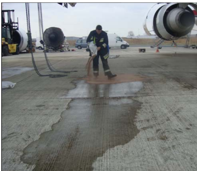
Figure 21: The use of absorption granules after spillage
