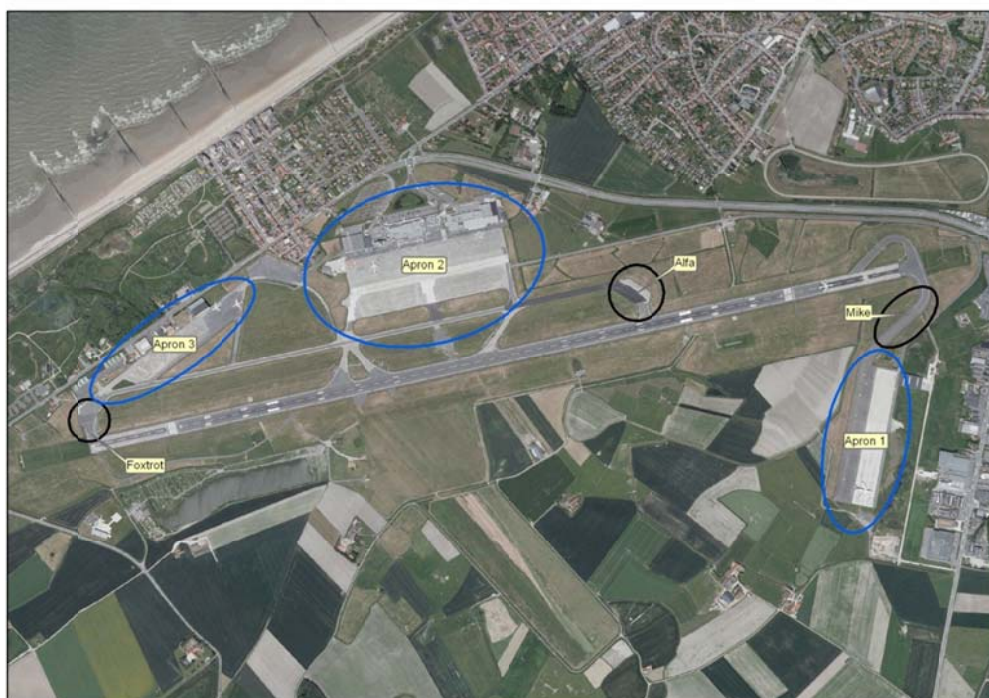
Figure 30: Overview of the aprons and locations for full power testing at Ostend Airport
